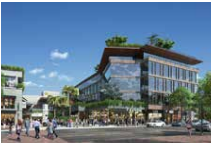
ONE COCOWALK 3001 Grand Avenue 79,930 SF Class A Office Developers: Federal Realty Investment Trust, Grass River Property LLC, Comras Company Delivering 4Q 2019
